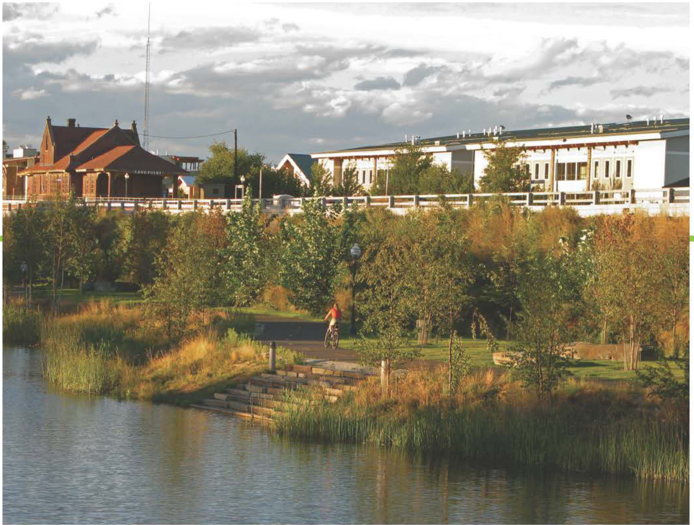
ABOVE: Sandpoint, Idaho brought in artist Vicki Scuri in 2000 to help design a highway bypass site. She found the community wanted a green wall. It was completed in 2012. OPPOSITE: The mechanically stabilized earth (MSE) green wall.
